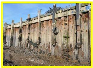
Corrosion and vegetation growth on steel sheet pile wall. (/1301C12)
