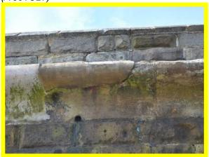
One remaining section of damage to the Previous repairs to the bullnose wave deflector bullnose wave deflector (/1301C27)
