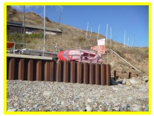
Missing coping at northern end of sheet pile wall (/1601C03).
