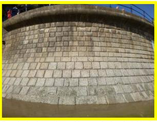
Historic horizontal cracking and abraded blocks (/1602C05)
