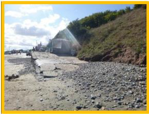
Toe of MU27/X showing signs of some localised recession adjacent to the Filey sea defences increasing the risk of outflanking.
