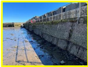
Local abrasion, cracking and spalling inside face of South Breakwater (/0403C03)
