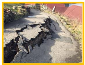
MU22/4 large cracks in footpath above chalets MU22/4 slope stabilisation works ongoing in the location of the wall failure (Photo from 2018 Report).
