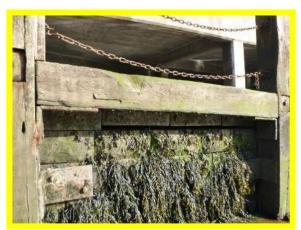
Minor damage and displacement to blockwork wall (/1301C14)
