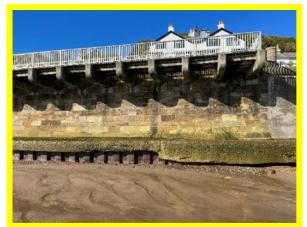
Toe structure undercut below masonry blockwork sea wall with cantilevered footway (\D0702C04)
