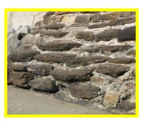
Typical defects (gaps) on blockwork wall (/1003C06)
