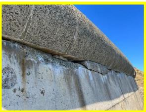
Abrasion and cracking of concrete coping (/0601C01)
