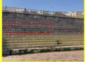
Concrete blockwall wall with buttresses (/1201C08)
