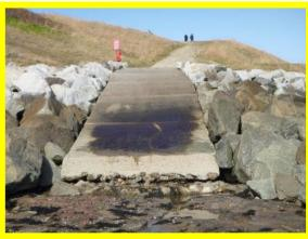
Vertical drop and crack in concrete at end of access ramp at south end of revetment (/1304C01)
