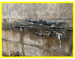
Surface cracking/abrasion (/0601C01)
