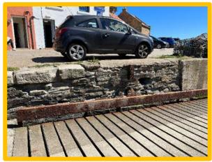
Poor condition masonry wall to rear of slipway (/0402C03)
