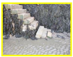
Access steps at root of East Harbour pier in poor condition. (/1301C01)
