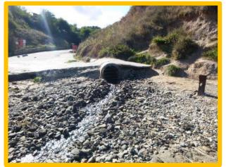
Undermined concrete access ramp and outfall between MU29/AI and MU29/AJ
