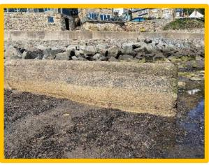
High beach levels obscuring undercutting identified in 2018 (/0601C02)
