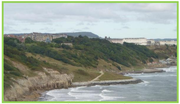
Rock revetment around debris lobe of Holbeck Hall landslide (/1304C01)
