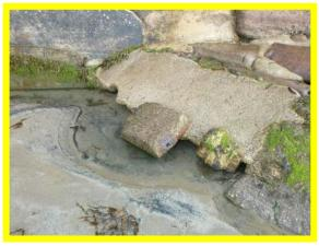
Undercutting of slipway toe and damage to previous repairs. (/1003C05)
