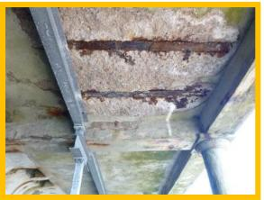
Damage to underside of upper promenade (/1302C01)
