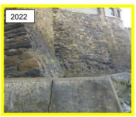
Typical defects (cracking) on toe (/1003C06)
