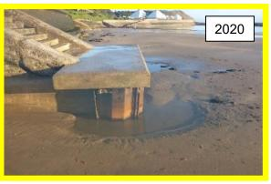
Corroded sheet Piles with minor seaward visible in 2020 (/1201C24)
