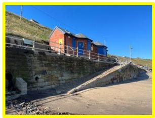
Masonry seawall and slipway in front of RNLI station (\D0802C13)
