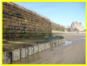
Masonry sea wall with exposed piles at The Spa access steps in fair overall condition (/1301C27)
