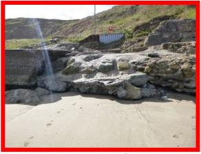
Voiding and undercutting of structure at the interface between (/1402C04) and (/1402C06).
