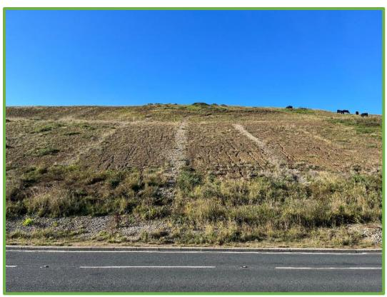
**MU9/3** Coastal slopes to rear of new sea defences generally in an inactive state following capital works involving re-grading, drainage and seeding as part of the Sandsend Road Coast Protection & Slope Stabilisation Scheme
