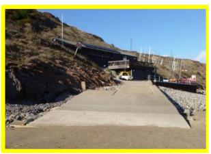
Some localised slumping of soft till onto upper section of slipway (/1601C03)
