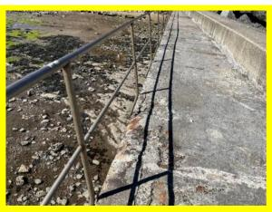
Abrasion to deck along inside edge of structure (/0402C01)
