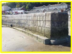
Undercutting at end of 'wing-wall' partially buried (/1602C09)
