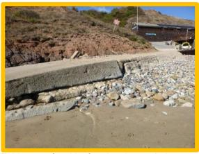
Evidence of voids forming beneath boatyard ramp (/1601C03)
