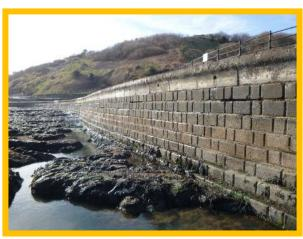
Previous repairs to wave return coping (/1303C02)
