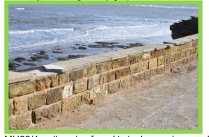
MU22/4 wall coping found to be loose, damaged MU22/4 – Inactive in 2022. and missing in places.
