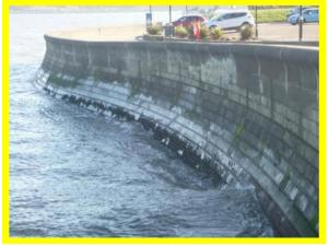
Fair condition seawall at Sea Life Centre Cracking in crest wall (/1201C02) (/1201C02)
