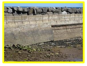
Detail on potential undercutting (left) and opening of construction joint (right) (/0402C01)
