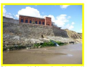
Private sea wall in fair overall condition but with the concrete apron is subject to ad hoc repairs in varying condition (/1402C05)
