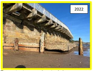
Toe structure undercut below masonry blockwork sea wall with cantilevered footway (\D0702C04)
