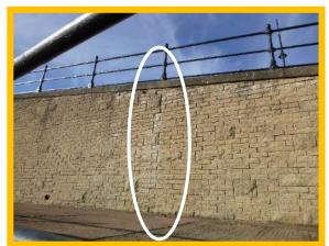
Original vertical crack in wall above access New vertical crack (/1301C10) ramp (/1301C10)
