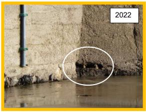
Spalling and loss of render in south face of West Pier wall. Void remains unchanged (/1301C07)
