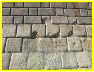
Occasional open joints with missing mortar and evidence of ongoing abrasion (/1602C06)
