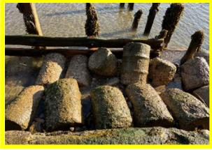
Displacement of some parts of the toe structure (\D0702C01)
