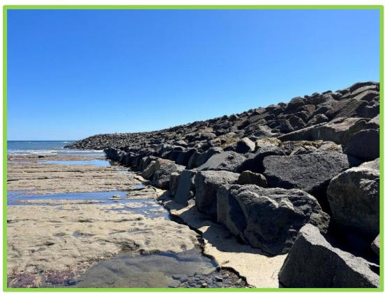
Rock armour revetment on seaward face of North Breakwater (/0402C01)
