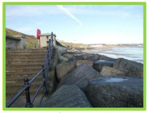
Rock revetment fronting seawall remains in good condition (/1202C01)
