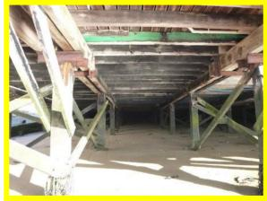
Low masonry wall underneath overhanging wooden promenade. (/1301C02)
