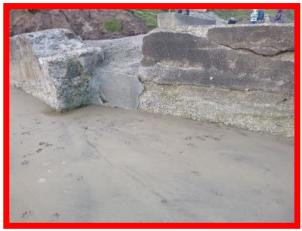
Concrete skim repair has filled voids and cracks (/1402C06)
