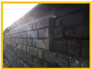
Repairs to wall face and coping in good condition. Extensive abrasion of adjacent blocks (/1302C02)
