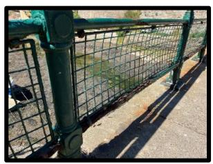
Footbridge – significant corrosion of bottom rail (no asset ref).
