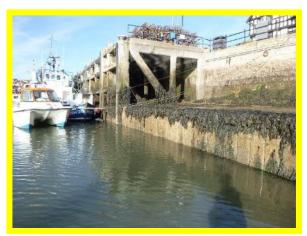
Suspended deck of concrete jetty (/1301C06)
