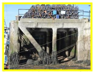
Suspended deck of concrete jetty (/1301C06)
