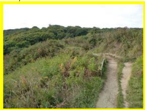
Headscarp recession has encroached on footpath. Note temporary boards to stabilise and mark path edge MU23/F.
