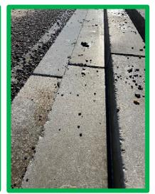
Loss of foam strips, abrasion to the toe beam, and at the leading edge of some stepped units
