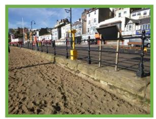
Beach levels flush with promenade at north end An area of abrasion at top of wall (/1301C23) of Foreshore Road seawall (/1301C15)
