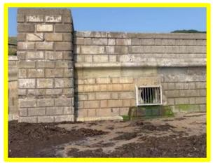
Area of recent repairs around outfall and to Missing blockwork in rear wall (/1201C04) promontory wall (/1201C04)
