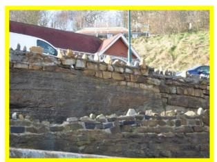
Overall fair condition of low stone wall. Overall fair condition of low stone wall and Damaged section of crest wall visible in centre access steps (/1302C03) of image(/1302C03)
