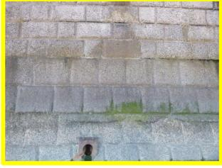
Example of replaced section of block work. Concrete repair undertaken with patterned shuttering to achieve blockwork effect (/1602C03)
