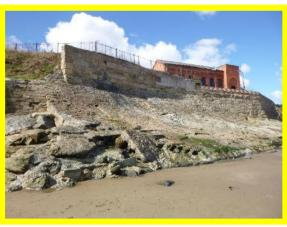
Evidence of voiding and deteriorations of grouted revetment at southern end of defence (/1402C05)
