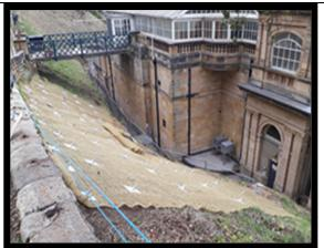
**MU22/2** Soil nail and slope mesh installation behind main Spa building in 2018
