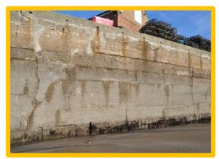
Longitudinal cold joints in south face of West Pier wall (/1301C07)
