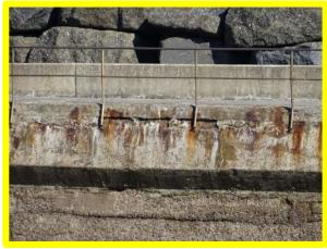
Rust staining and opening of construction joint on inside face of structure (/0402C01)
