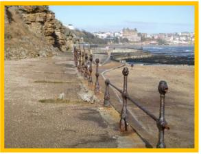
Upper prom has been fenced off and is in poor condition, heavily abraded and damaged handrail (/1304C02)
