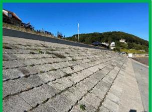
Coastal defences at Sandsend Road showing stepped pre-cast apron and upper Dycel units (\D0702C02)
