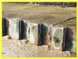
Corroded sheet piling along concrete apron(/1301C27)
