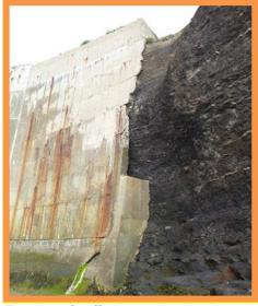
Erosion of cliffs immediately adjacent to large northern end of large sea wall (/1003C03)
