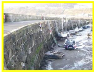
East Harbour inner pier, historically repaired joints visible (/1301C16)
