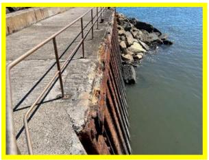
Significant corrosion / loss of section of sheet piles (/0402C01).
