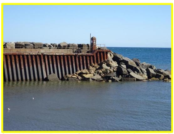
Corroded steel sheet piling on inner face of North Breakwater. Rock armour profile appears similar to 2020 inspection (/0402C01)
