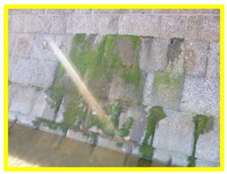
Abrasion damage and several leaking joints (/1602C03)
