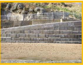
Seawall in overall poor condition Cracks to bastion throughout. Mortar missing between blockwork in lower wall. (/1304C02)
