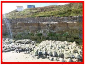
Missing mortar and damaged blockwork (/1402C04)
