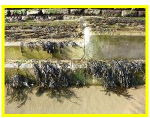
In front of the Sun Court (/1301C28), the wall has a concrete 'nosing' intended to act as a wave deflector below the parapet. Previous repairs to this element remain effective. There was one new section of damage noted on the wave deflector nosing. It is recommended that this is repaired. The concrete toe beam was partially exposed along the length of the Sun Court and visible sections appeared in fair condition.
