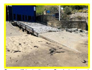
Former lifeboat slipway. Beach levels and seaweed largely obscure previous repairs/concrete pours at the toe (/1003C04)
