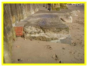
Abrasion of toe apron south of previous repairs beach levels notably higher than 2018 (/1301C09)
