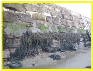
Open joints at base of wall, principal blockwork appears in fair condition (/1301C16)
