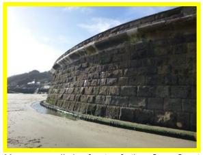
Masonry wall in front of the Sun Court. Concrete toe partially visible (/1301C28)
