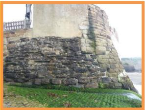
Blockwork wall in poor condition fronting the Bay Hotel (/1003C04)
