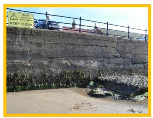
Large open joints and cracks are evident from timber piles visible at toe of wall (/1301C07) along the wall's full extent (/1301C19)
