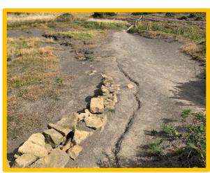
MU15/2 Tension cracks on access path to the south of Far Jetticks
