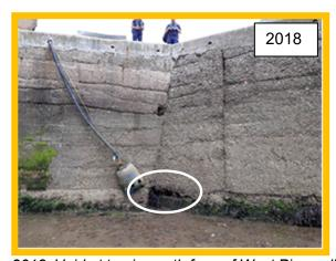
2018: Void at toe in south face of West Pier wall and damaged conduit (/1301C07)
