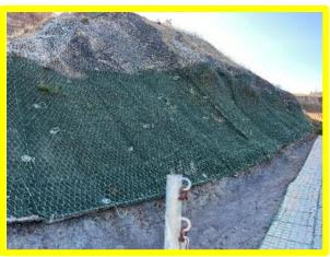
Slope protection netting above the access ramp (\D0803C05)
