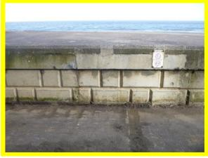
Vertical crack (seen from rear of crest wall) (/1201C06)
