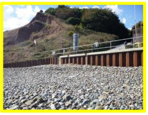
High shingle levels conceal much of the sheet pile wall (/1601C03).
