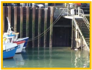
Corroded steel sheet piling notably worse directly adjacent slipway (/1301C13)
