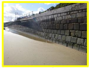
Previous repairs to crest of slipway 'wing-wall' (/1602C09)
