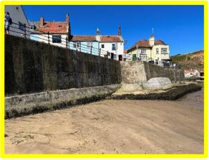
Abrasion and cracking to seawall face and crest at interface between different wall sections (/0403C05)
