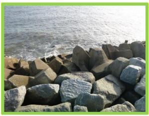
Example of locally cracking and movement of Accropode units, but otherwise revetment in good condition (/1202C02)
