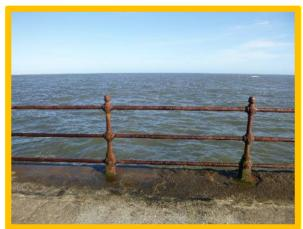
Heavily corroded handrail (/1201C03)
