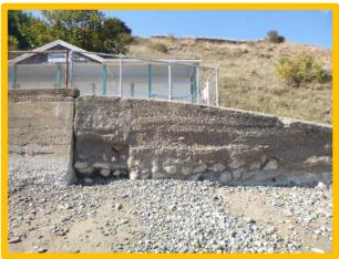
Heavy Abrasion damage to the rear wal (/1602C01)
