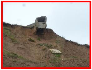
Looking from up from the beach at the base of MU24/M1 in September 2018, note undercutting of Pill Box.
