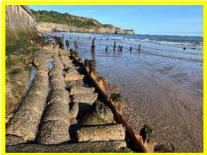
Toe structure formed from concrete-filled barrels (\D0702C01)
