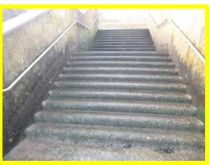
Heavily abraded steps with rounded edges (/1202C01)
