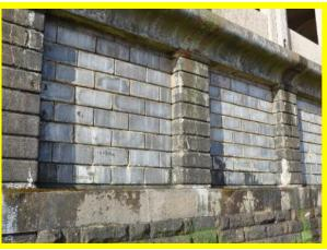
Repaired sections of beam in good condition (/1301C29)
