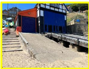
Open joints / cracks in Runswick Rescue slipway (/1003C04)
