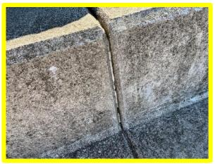
Brittle/missing flexible sealant from expansion joints (/0403C03)
