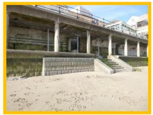
Repairs to lower wall at the open colonnade are in good condition with remaining sections of December 2013 storm damage (/1302C01) original wall in fair condition. (/1302C01)
