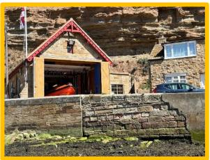
Potential void beneath un-rendered section of masonry wall (/0402C03)
