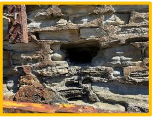
Missing blockwork in masonry wall to rear of slipway (/0402C03)
