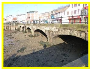
Some Cracking and missing joints to capping apron to wall south of roundabout opposite arcade. (/1301C05)
