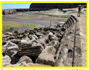
Lower crest level at northern extent of rock Southern extent of rock revetment (/0402C02) revetment (/0402C02)
