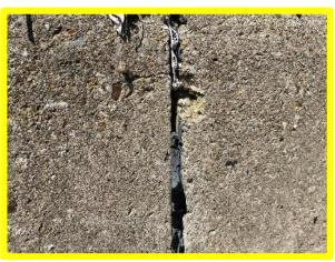
Brittle/missing sealant in expansion joints (vertical and horizontal). Vegetation growth locally. (/0601C03)
