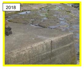
Typical defects (cracking) on toe apron (/1003C06)
