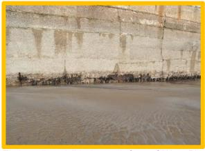
Timber piles visible in south face of West Pier wall (/1301C07)
