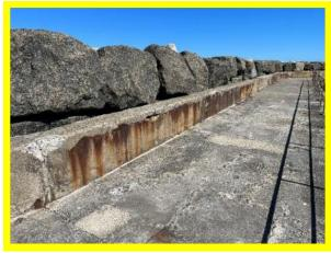
Crack, abrasion and rust staining of crest wall (/0402C01). No significant change from 2020.
