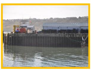
Corroded steel and damage to capping beam on inner face of West Pier (/1301C1718)
