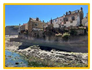
Variety of masonry and concrete walls. Vegetation growth locally (/0402C04)
