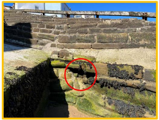
Void at interface between sea wall and south face of slipway (/0403C05)
