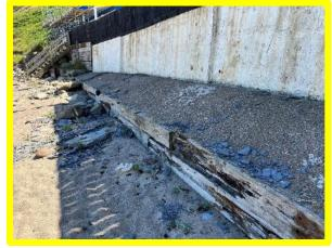
Rotten/missing timber (permanent formwork for Crack in concrete wall (/0602C05) concrete behind) (/0602C05)
