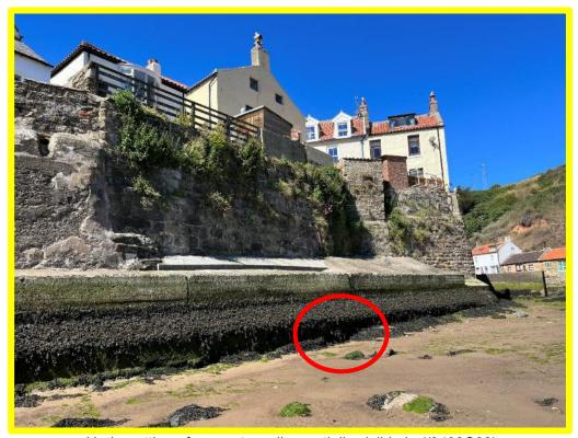
Undercutting of concrete wall – partially visible in (/0402C22)
