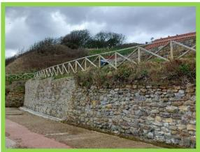
MU22/4 - recently completed retaining wall (left) transitioning into repointed pre-existing masonry retaining wall (right)
