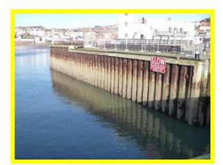
Corroded steel sheet piling (/1301C17)
