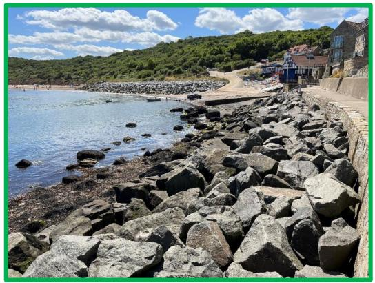
Rock armour fillet at toe of existing seawall, seed rocks seaward of toe as constructed, July 2022.I
