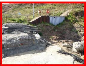
Undermining of footpath beneath 'Lucy's Shack' (/1402C04)
