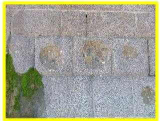
Example of 'pockmark' abrasion pattern which is common along the Filey Seawall (/1602C03)
