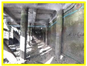
Abrasion to quay wall beneath suspended deck (/1301C06)
